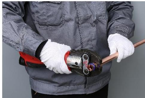
Press jaws must be positioned at right-angle to the joint to ensure even pressing pressure is applied.
